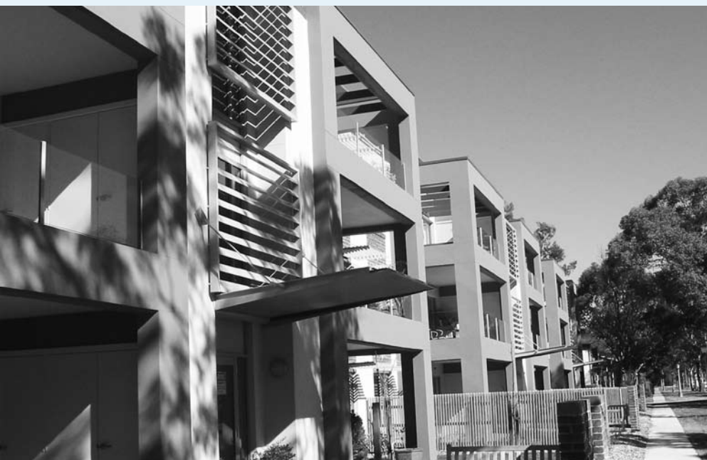
Accessible housing for older people in Turner.
